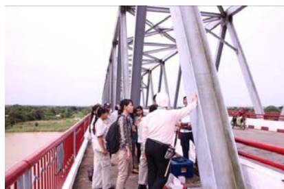
Investigation of Moubin bridge
