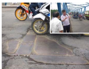
Photograph 3: Bridge pavement evaluation in Bandung
