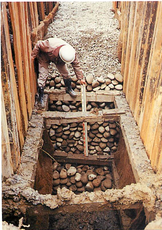
▲ 3号排水壁工施工中 Under construction of No.3 Pervious wall
