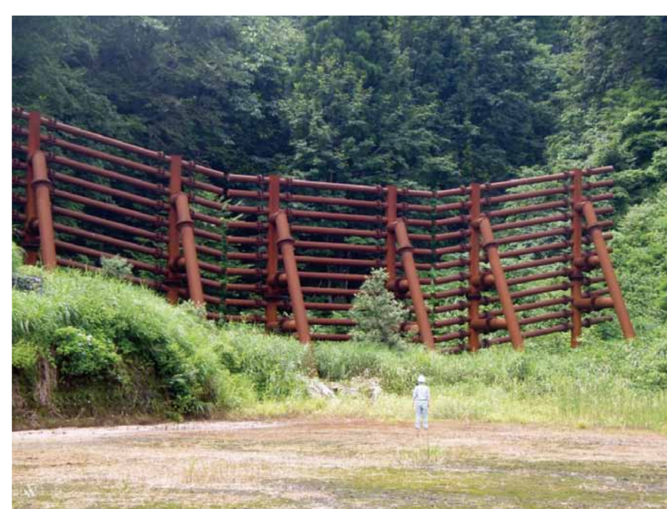
▲ 雪崩防護柵(阻止工) (新潟県柏崎市) An avalanche protection structure (defensive structure) (Kashiwazaki City, Niigata)
