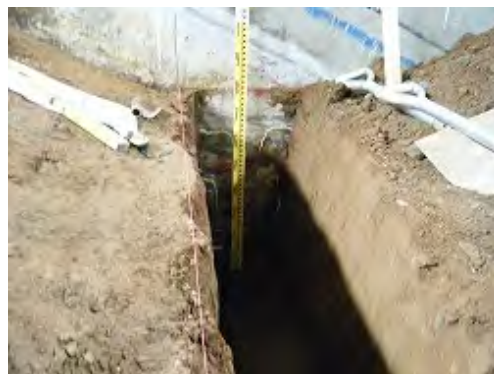
(b) 掘削深さ確認
